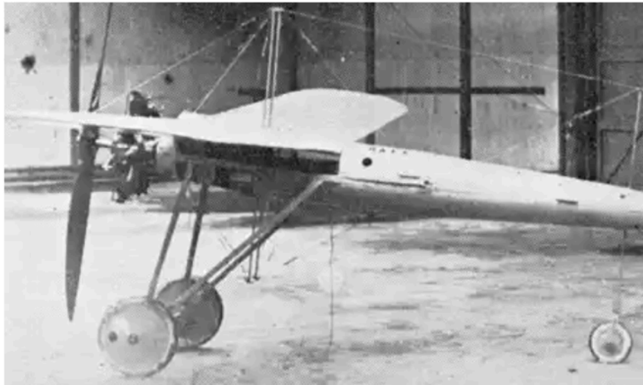
Figure 3. Early UAV design, called Aerial Target 1916 [58]
